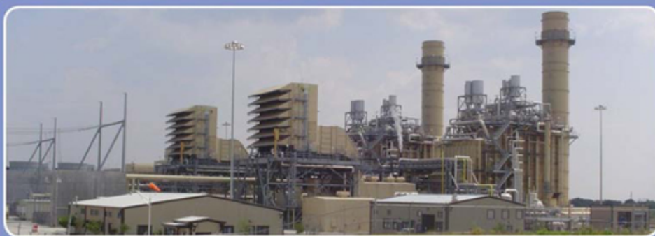
Wolf Hollow is a 720 megawatt combined-cycle natural gas-fired power plant located in north Texas.
