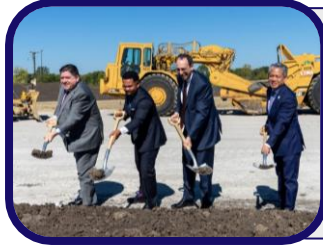
September 13, 2024 IL: CyrusOne Aurora Data Center
